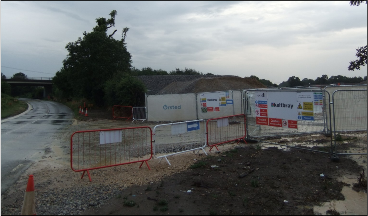
Figure 3: View looking north
